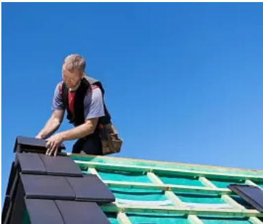
District Of Columbia Roof Replacement Costs Might Surprise You RoofReno
